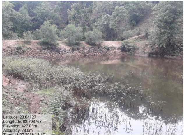
Earthen dam in the downstream
