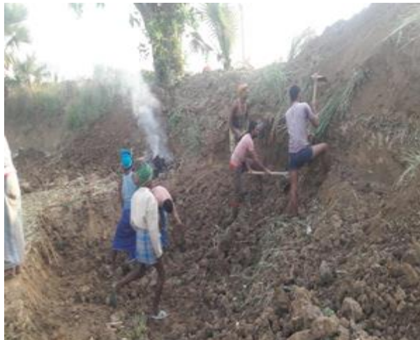
Villagers of Saidpur repairing damaged pyne wall
