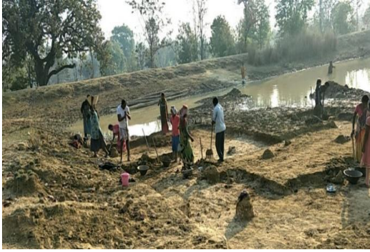
Initiation of earthen embankment and deepening of pond
