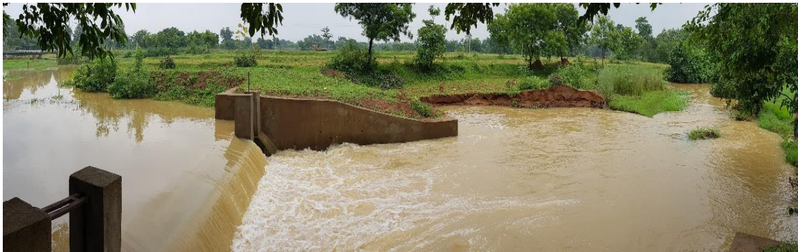
Completed check dam as recommended by ICRG programme in Dudhiasole village – OAIC will facilitate lift irrigation at this site
