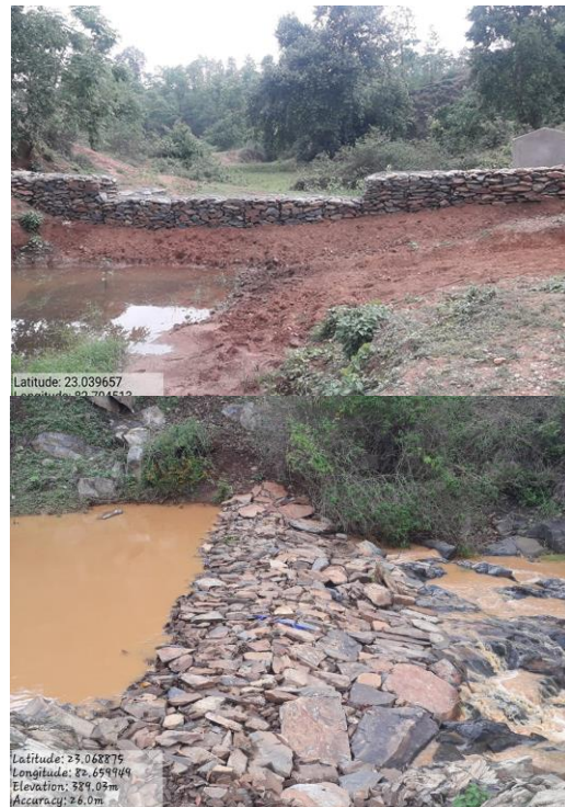
Climate Resilient Work – Gabion and Loose Boulder Check Dam
