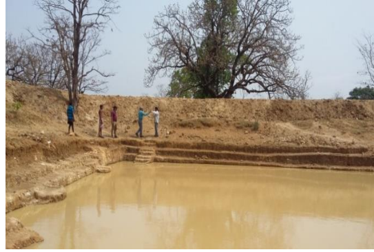
Initiation of earthen embankment and deepening of pond
