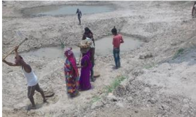
Pond rejuvenation work in progress in Barri gram panchayat
