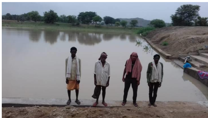
The tank filled with water
