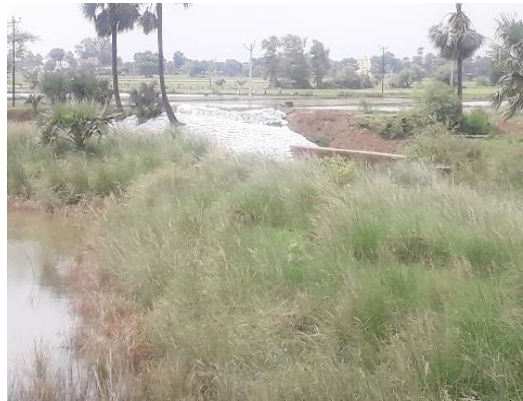
Repaired Chilkha in Diyawan
