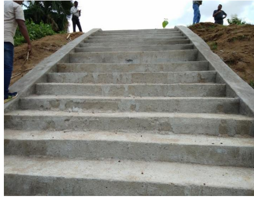
Construction of bathing steps using 14 th Finance Commission funds
