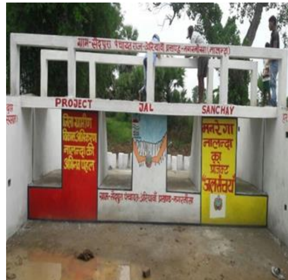
Completed check dam at suitable site
