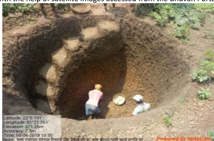
Construction of recharge pit in progress
