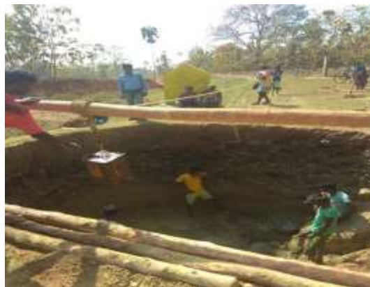
Construction of dug well
