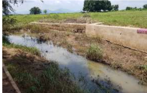
Check dam remained undamaged even after overspill of water
