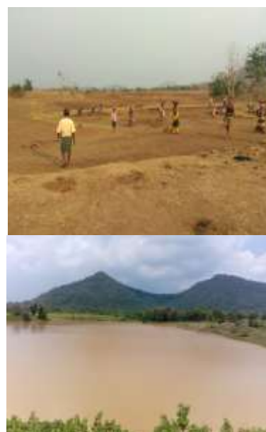
Renovation of water harvesting structure
